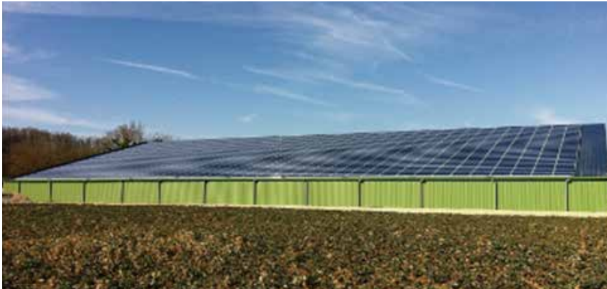
France Grosdenier 243 KW Rooftop Project
